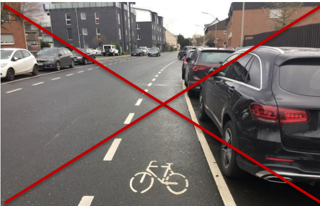
Figure 12: Requirement of safety clearance between parking and cycling in mixed traffic with and without advisory lanes according to the RAST fact sheet of R Climate (example, own photo, own illustration).
