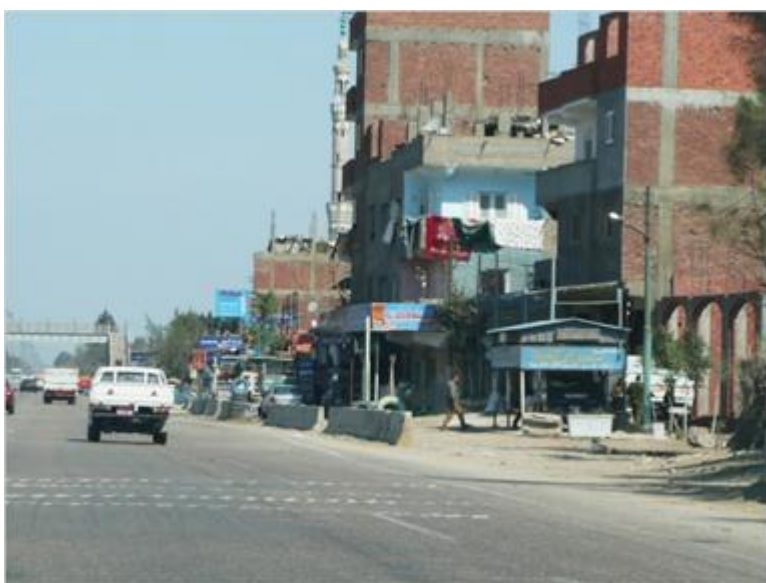
Figure 8: Example of a Motorway through urban areas without access control (Cairo-Alexandria Desert Road in Egypt)
